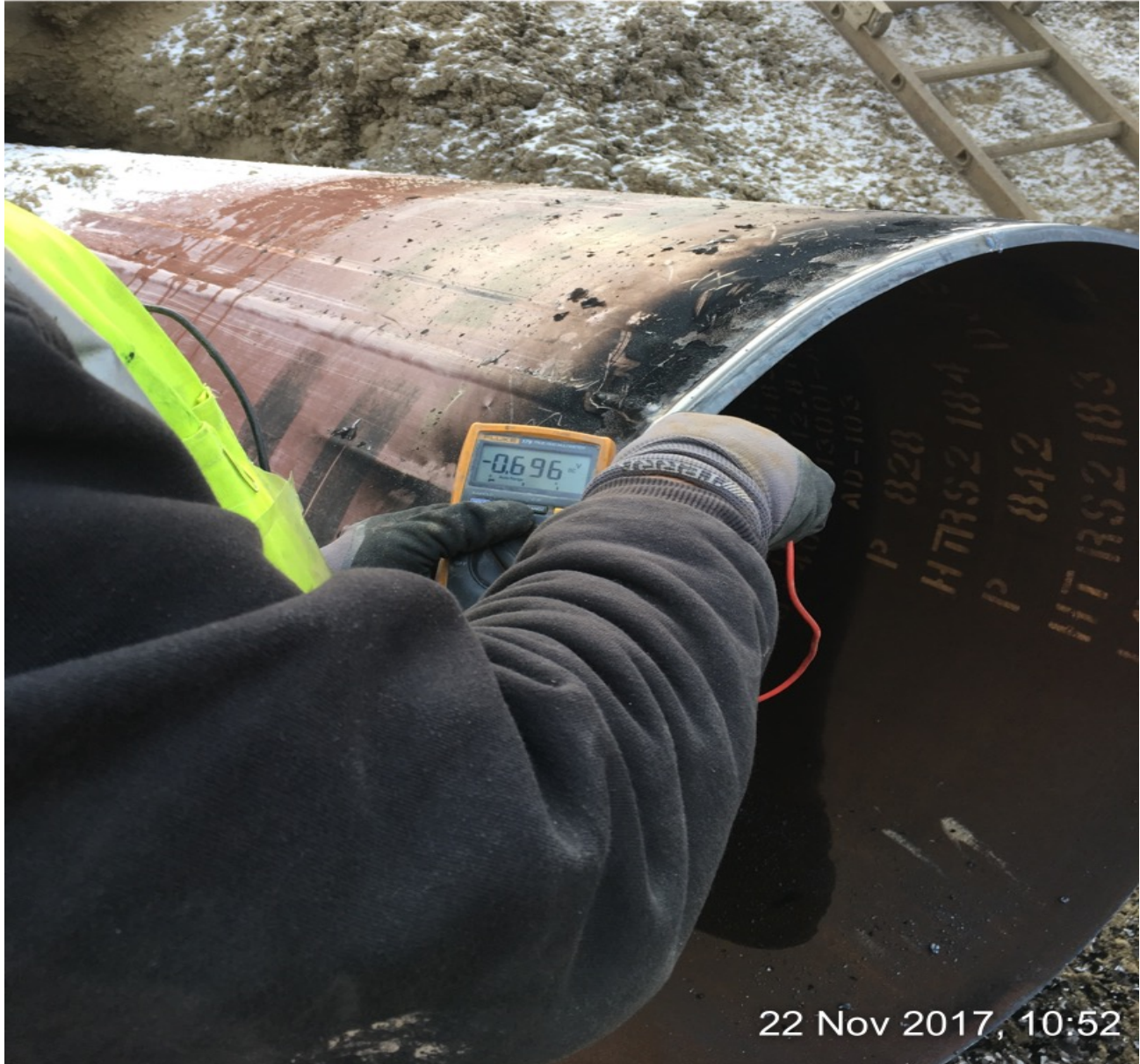
CORRISION TESTING ON PIPE THAT WAS PULLED FROM UNDERNEATH A ROAD
