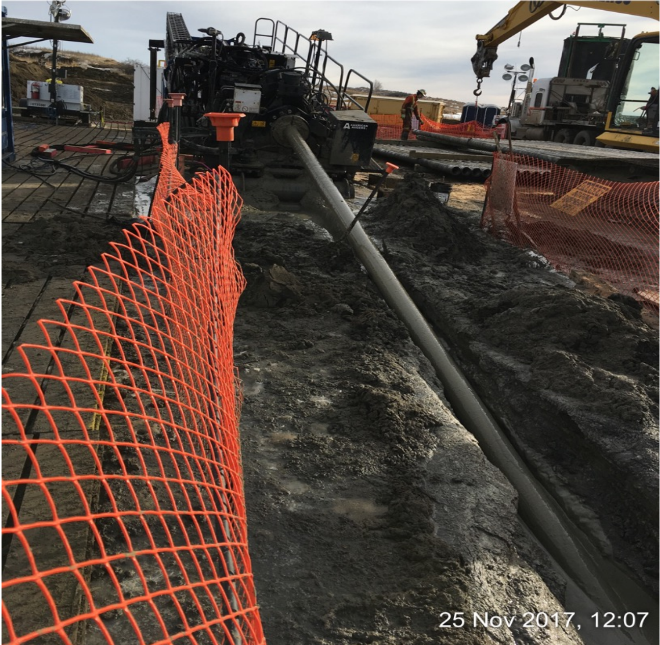
EXIT POINT OF HORIZONTAL DIRECTIONAL DRILLING
