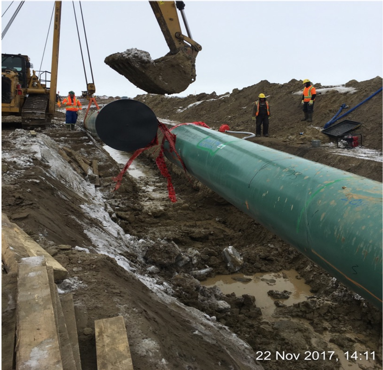
CREW WORKING ON A TIE IN
