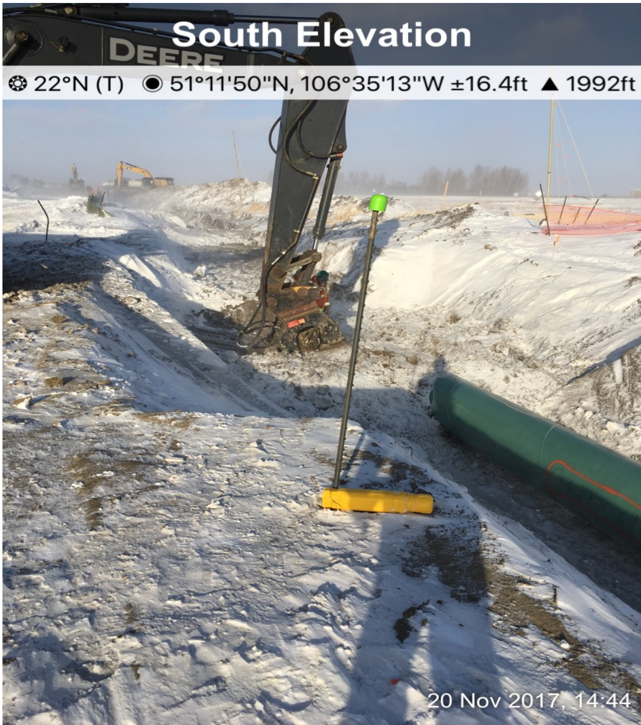
HOE PACKING OF BACKIFF SOIL
