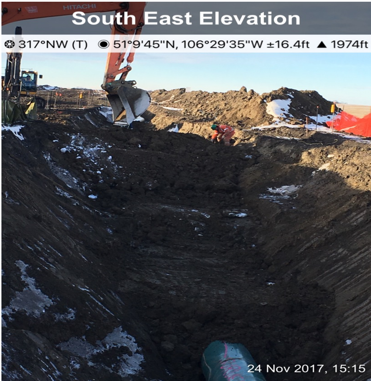
BACKFILLING AND PACKING SOIL ON HOTLINES
