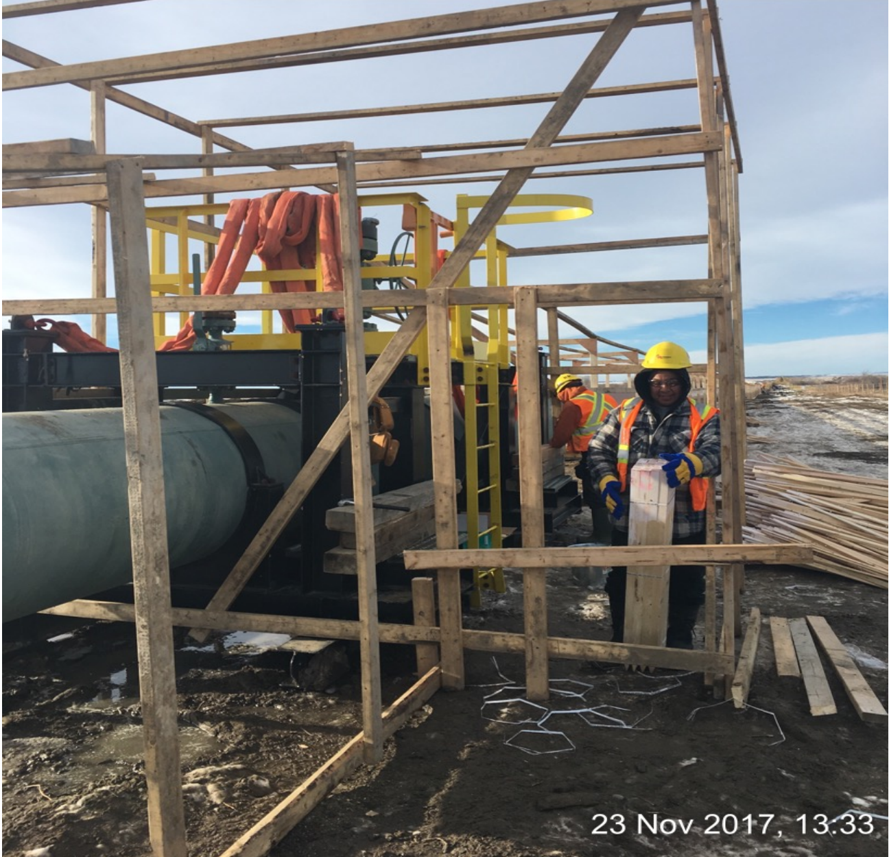
CREW WORKING ON HOARDING THE PIPE
